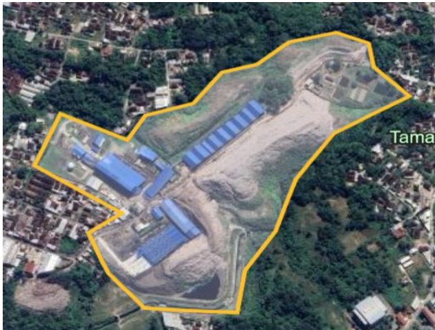
Figure 6. Location of the Putri Cempo Landfill and WtE Facility (110° 51' 21.74" E, 07° 32' 8.11" S)
